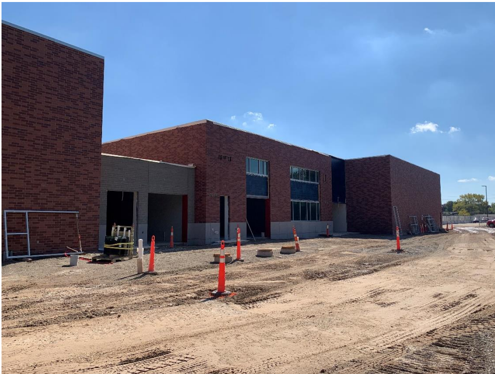
9. Area 2A & 3 East – Masonry is installed. Metal wall panel girt system and storefront glazing install in progress.
