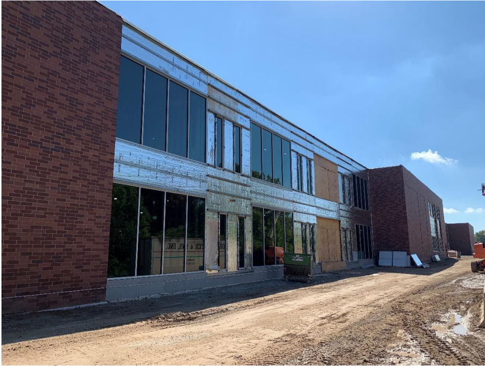
9. Area 2A & 3 East – Masonry is installed. Metal wall panel girt system and storefront glazing install in progress.
