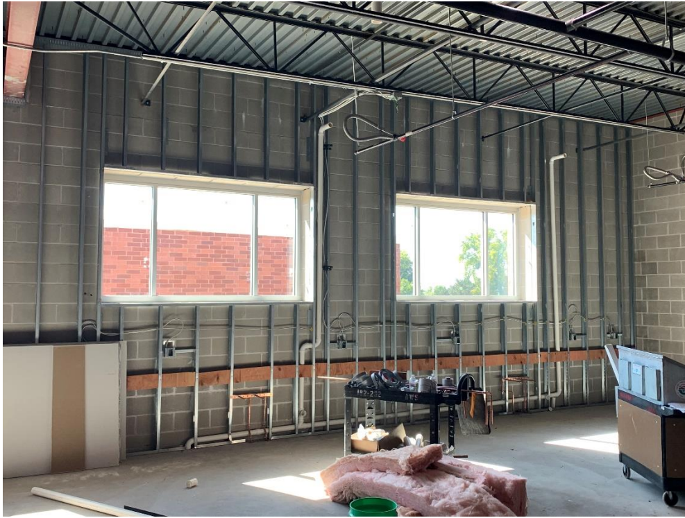
24. Area 3 – Exterior storefront installed. In wall plumbing and metal stud furring in progress.
