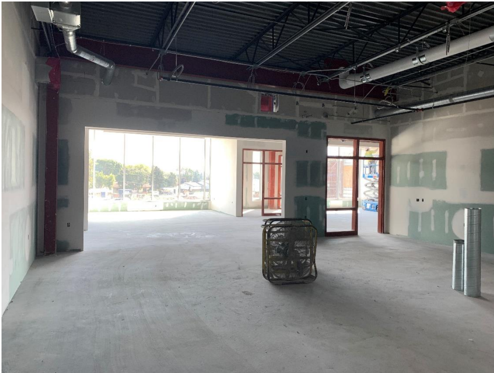
17. Area 5 - Above ceiling MEP installation and soffit cold form framing in progress.
