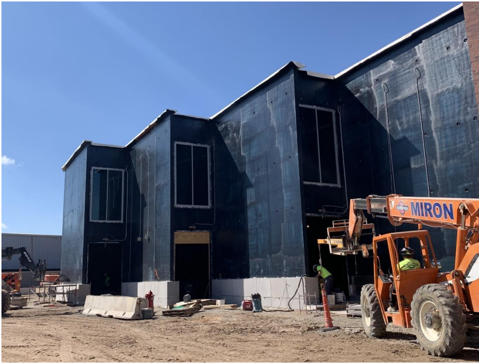
5. Area 6 North – Board insulation installed. Metal wall panel girt system, storefront glazing, and roof coping install in progress.
