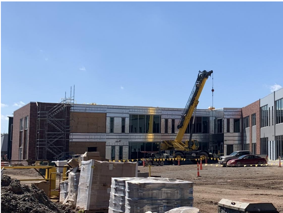
5. Area 6 North – Board insulation installed. Metal wall panel girt system, storefront glazing, and roof coping install in progress.
