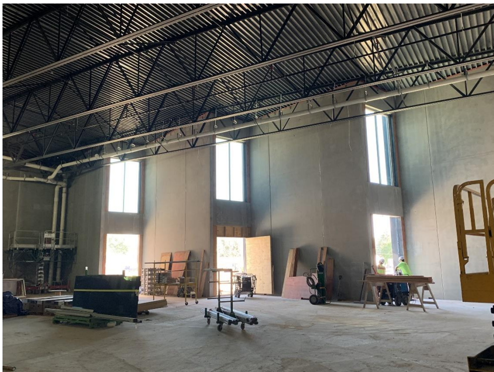
29. Area 6 – Install of exterior storefront at east gym wall in progress. Above ceiling MEP install in progress.
