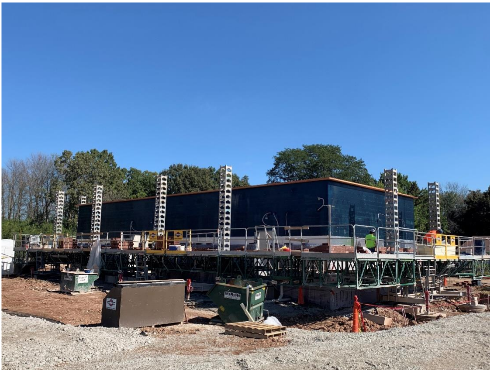
13. Locker room building masonry install in progress. Spray applied AVB and top of wall blocking installed.
