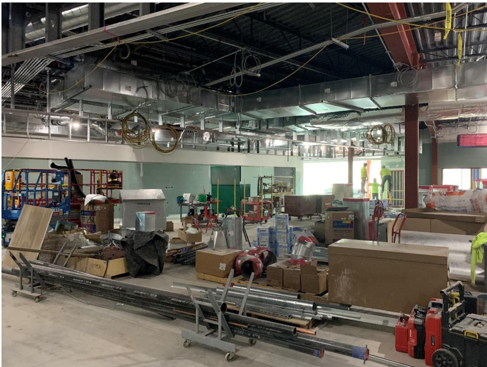
17. Area 5 - Above ceiling MEP installation and soffit cold form framing in progress.
