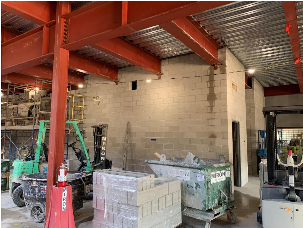
28. Area 1A – Interior cmu locker room walls are being laid.
