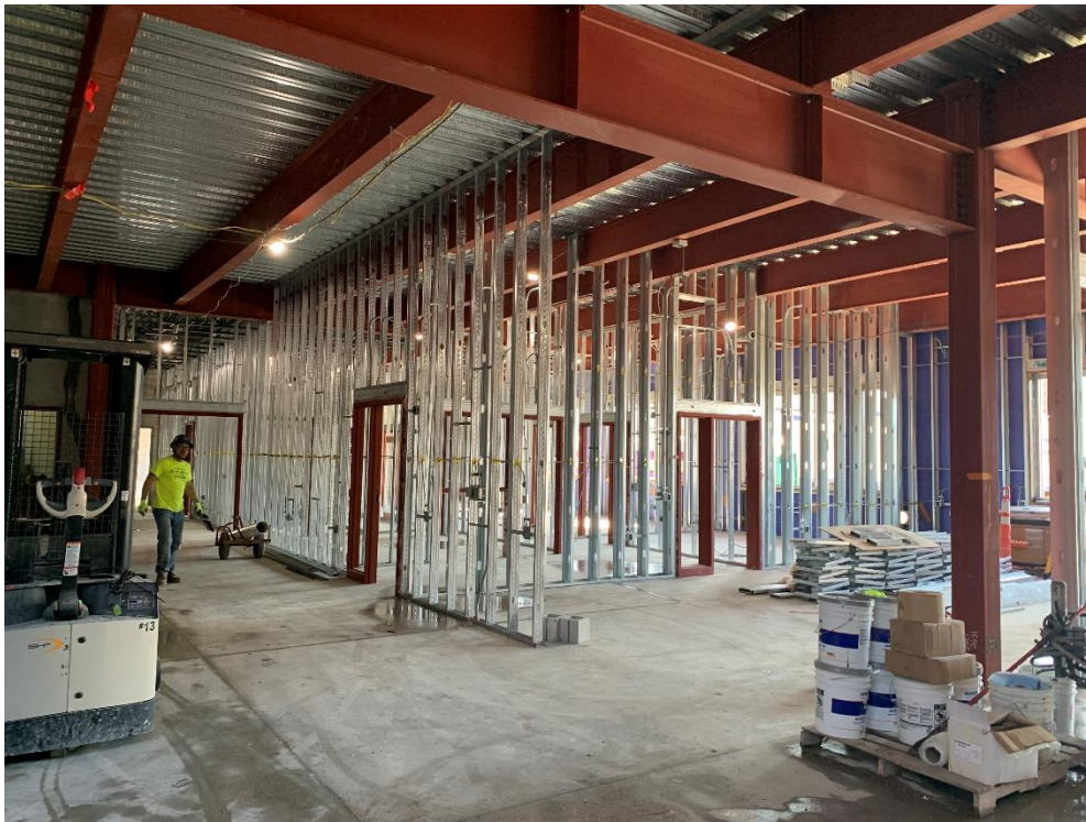
26. Area 1A – Interior metal stud wall framing install in progress at 7/8 school office area.
